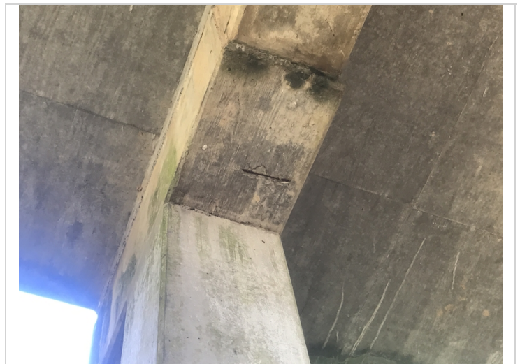
Bent 4 cap bottom has spall with exposed rebar.
