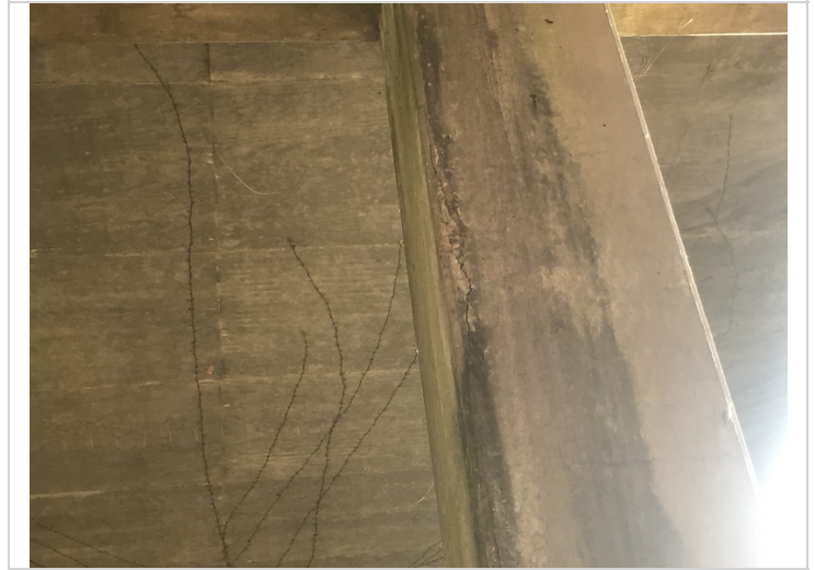
Bent 3 column 3 has delam.
