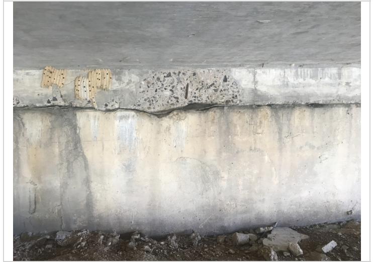
Deck haunch above bent 6 has spall with exposed rebar.
