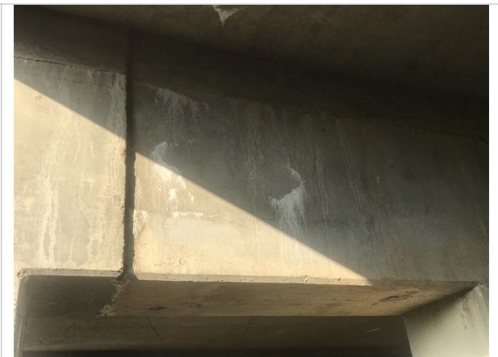
Bent 5 cap ahead has cracks with efflorescence.
