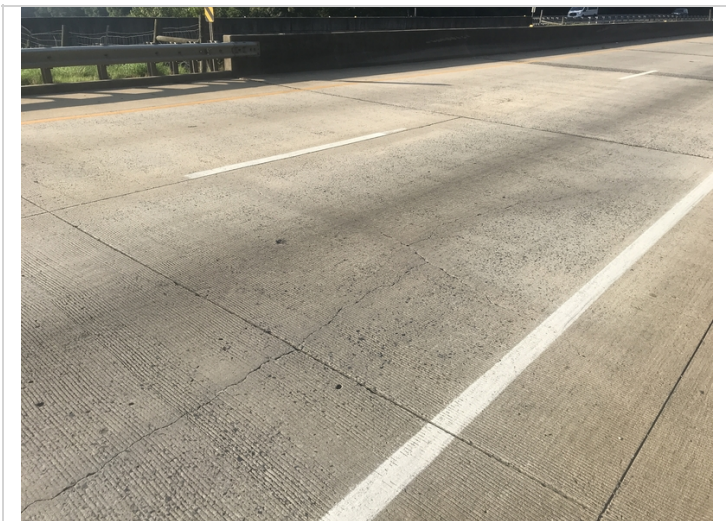
Large unsealed cracks in the east approach slab.
