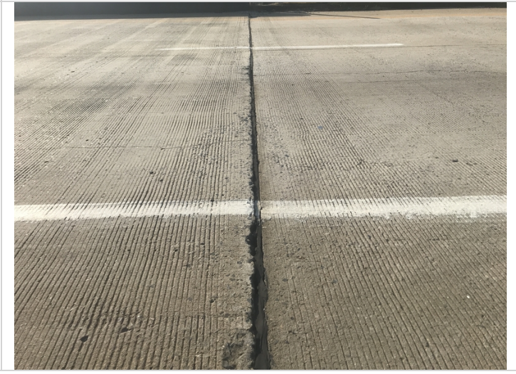
Bent 1 joint seal has lost bond and is leaking. Common all joint seals.
