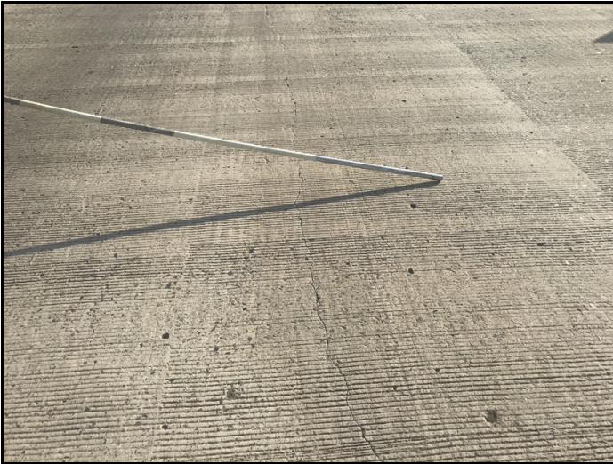
Span 5 deck has longitudinal crack that reflects through to the soffit at centerline.
