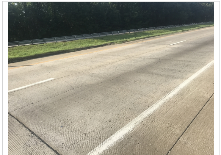
West approach slab has large unsealed longitudinal crack.
