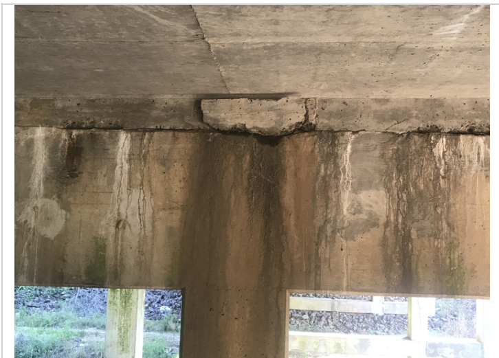
Bent 2 above cap haunch of deck has delam.
