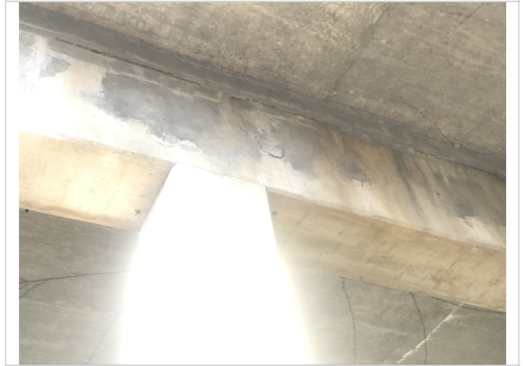
Bent 4 cap ahead has delam.
