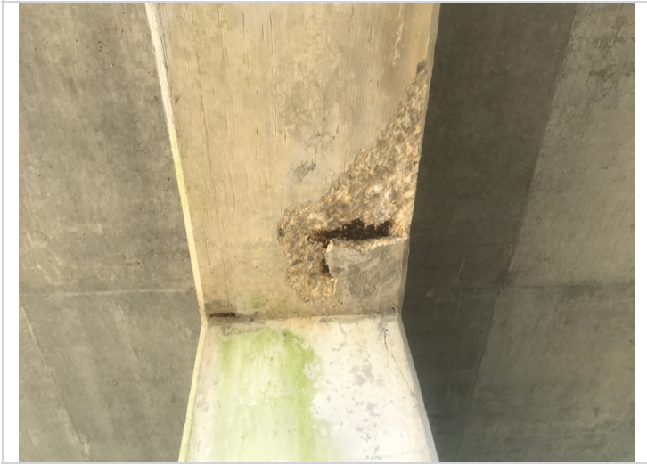
Bent 5 cap bottom has spall with exposed rebar.
