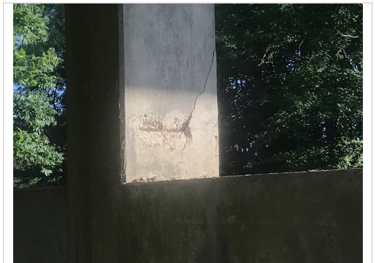
Bent 2 column 2 has spall with exposed rebar.
