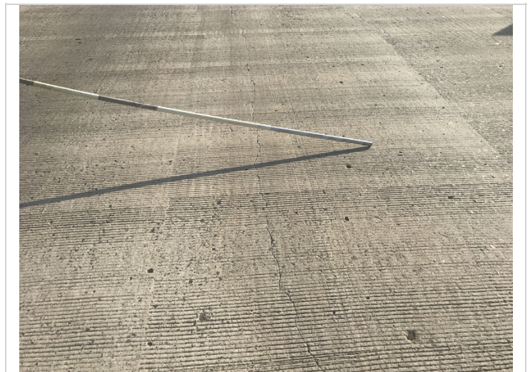
Span 5 deck has longitudinal crack that reflects through to the soffit at centerline.
