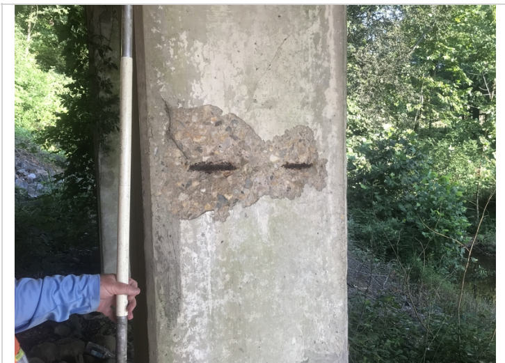
Bent 2 column 2 has spall with exposed rebar.
