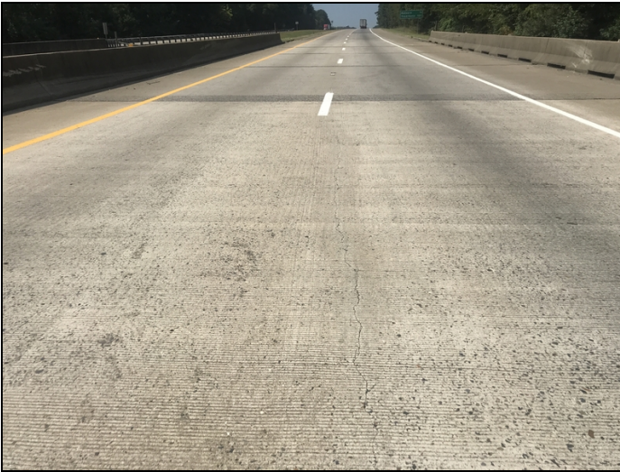
Span 5 large longitudinal cracks.
