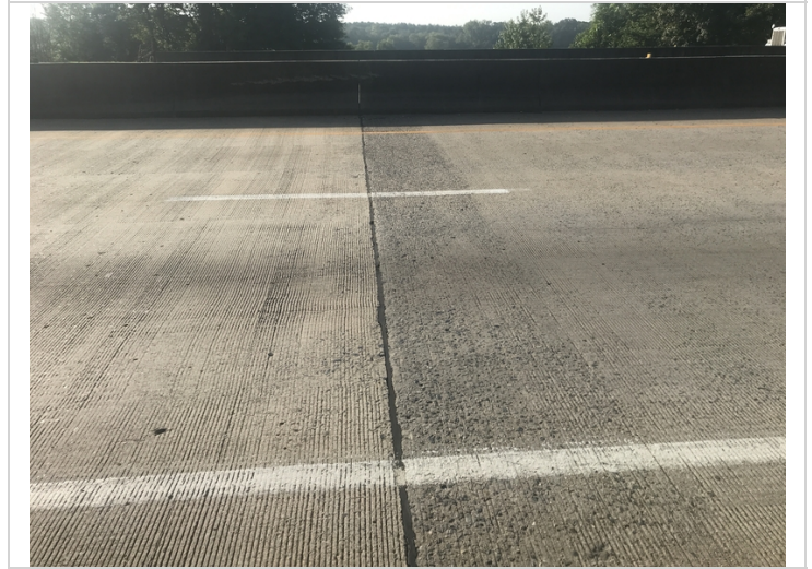
Span 4 at bent 5 deck has abrasion common bent 2.
