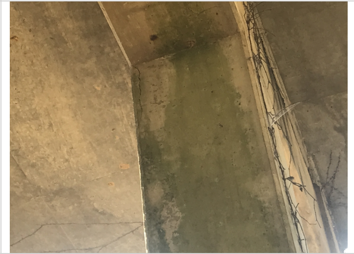
Bent 4 column 3 has large crack.
