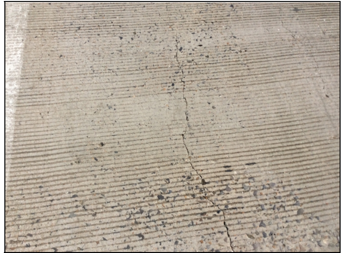
Deck has large unsealed cracks.
